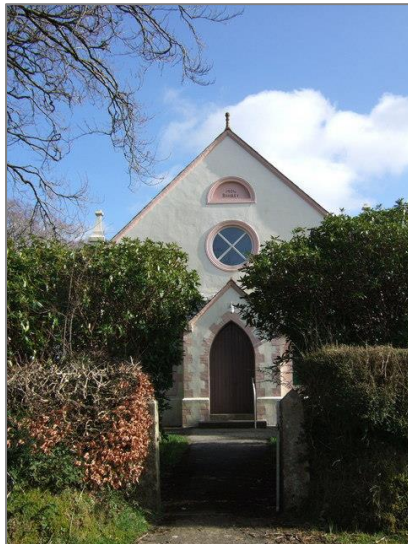
Figure 10. Boasley Methodist Chapel built in 1838 and re-built in 1904, still holding services today © Copyright Derek Harper, CCA
